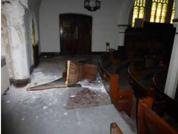
60. Broken pews and plaster columns (ERA, 2015).
