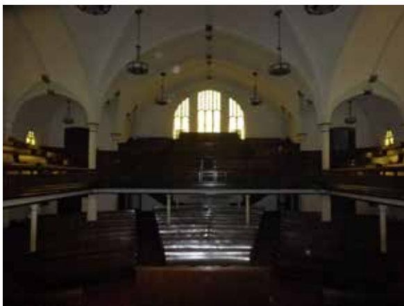
50. East elevation of the sanctuary (ERA, 2015).
