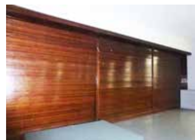
67. Wooden dividers that roll down from the ceiling (ERA, 2015).
