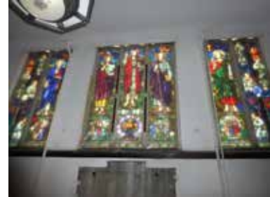
49. Stained glass windows, with evidence that a plaque or tablet has been removed from the narthex (ERA, 2015).
